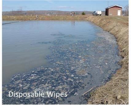
Wipes and hygiene products do not biodegrade, accumulate in the lagoon, and rot; odor.
